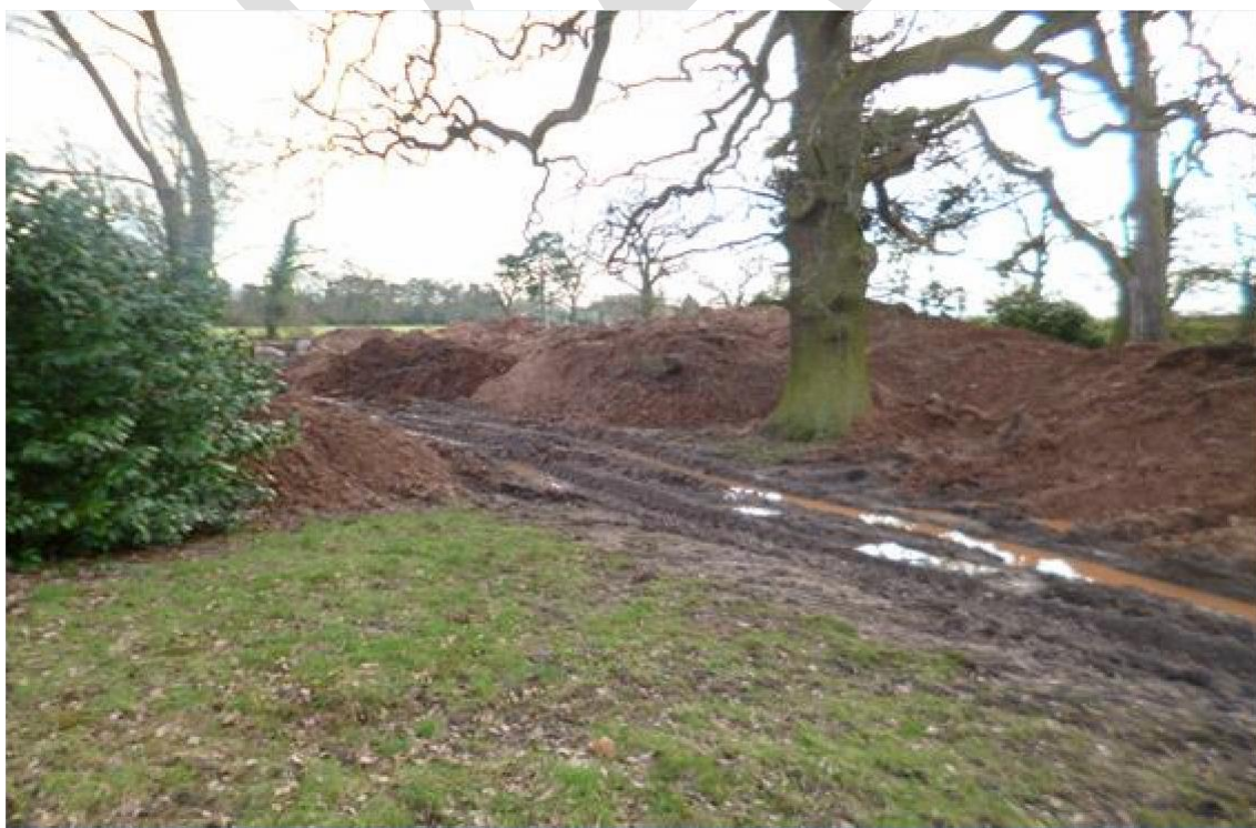
Damaged soil structure from the passing site vehicles within the Root Protection Zone.
